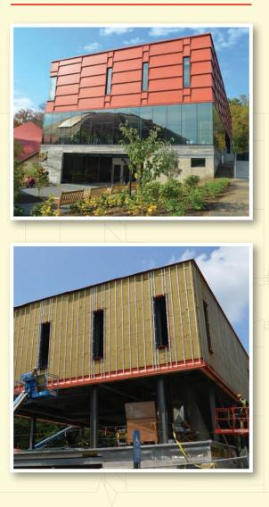
The Matchbox features three cladding systems stacked one on top of the other—rain screen over curtainwall over rubble-stone wall. The architectural firm, Philadelphia-based DIGSAU, wanted a system that would minimize thermal bridging while providing a rainscreen backup wall with attachment points at varying depths.
