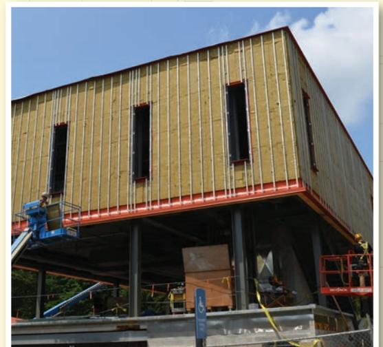
The Matchbox features three cladding systems stacked one on top of the other—rain screen over curtainwall over rubble-stone wall. The architectural firm, Philadelphia-based DIGSAU, wanted a system that would minimize thermal bridging while providing a rainscreen backup wall with attachment points at varying depths.
