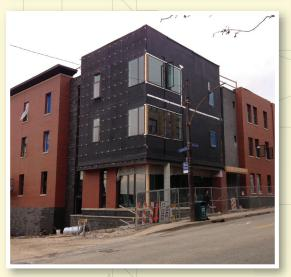
manufacturer and could be installed completely on the outside of the sheathing air barrier, maximizing the continuous insulation and minimizing thermal bridging.
