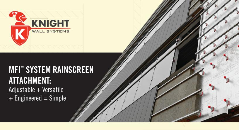
The Knight MFI™ System dramatically reduces the thermal bridging within rain screen systems using mineral fiber insulation, while providing limitless design options for building facades; combining energy efficiency, façade versatility, and long term sustainability.
