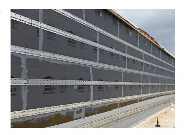
For basic, cost-effective vertical claddings, only a single layer of HCI-GIRT may be needed. For more complex cladding designs or types, choose from a wide variety of KWS™ secondary rails for those panels requiring specific attachment points.
